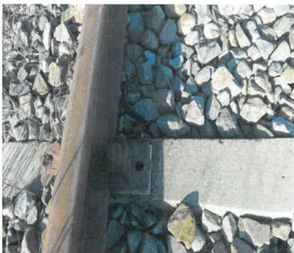
Inel resort lipsă, prinderi inactive
