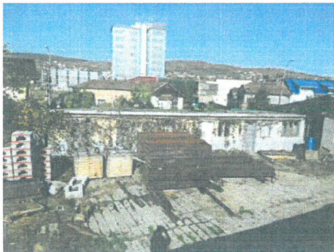
Statia Cluj – Cladire District Poduri L3
