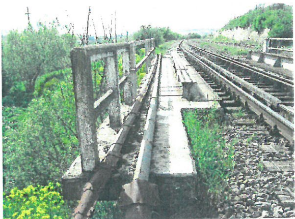
7. Parapet culee linia 2
