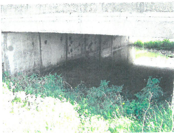
11. Elevatii prefabricate, culee Oradea
