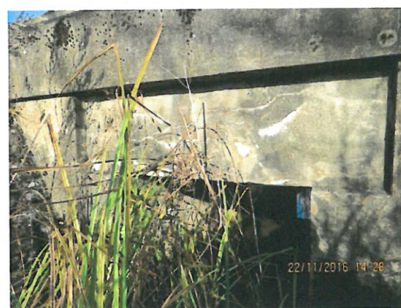
6. Detaliu timpan aval
