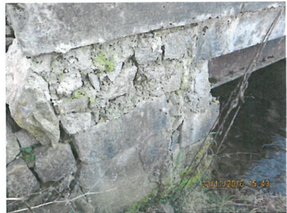
10. Detaliu timpan aval
