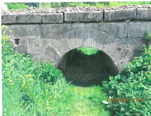
10. Detaliu timpan aval
