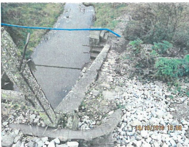
5. Scară acces culee Cluj, in aval
