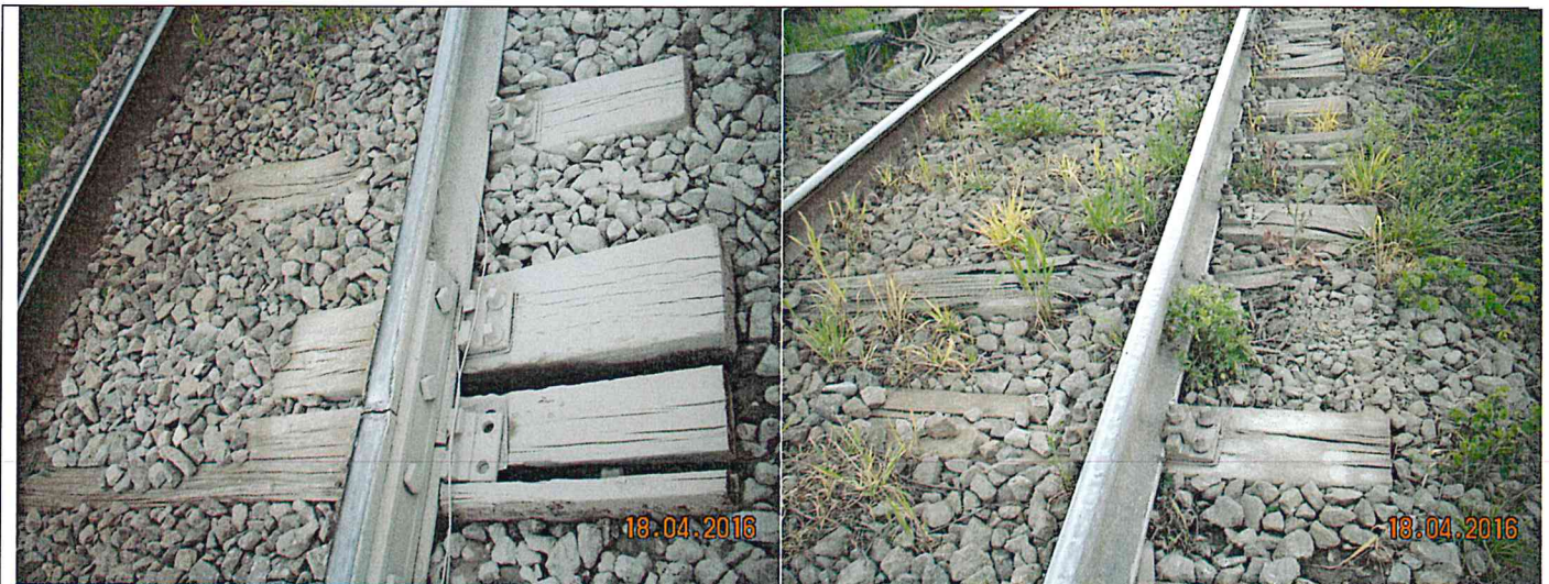
Traverse de lemn crapate, rupte, putrezite
