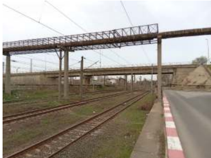
Figura 6. Supratraversare de conducte km 227+115,69 (topo)
