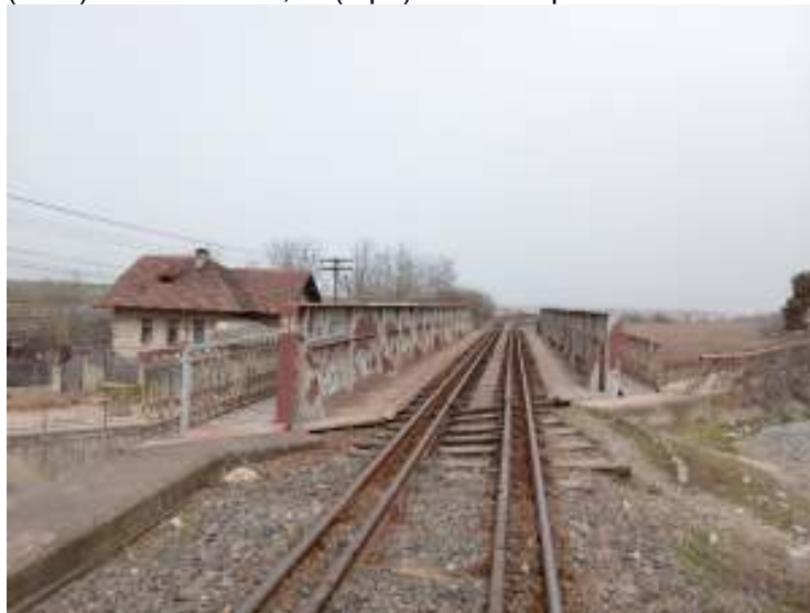
Figura 23. Pod km 244+715 (CFR) / km 244+678,55 (topo)
