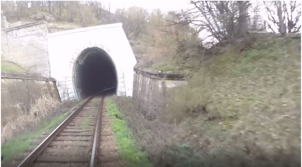
Figura 9: Tunel Bahna existent
