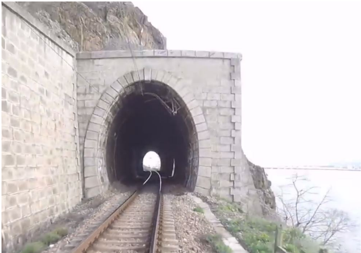
Figura 3: Tunel Baba existent
