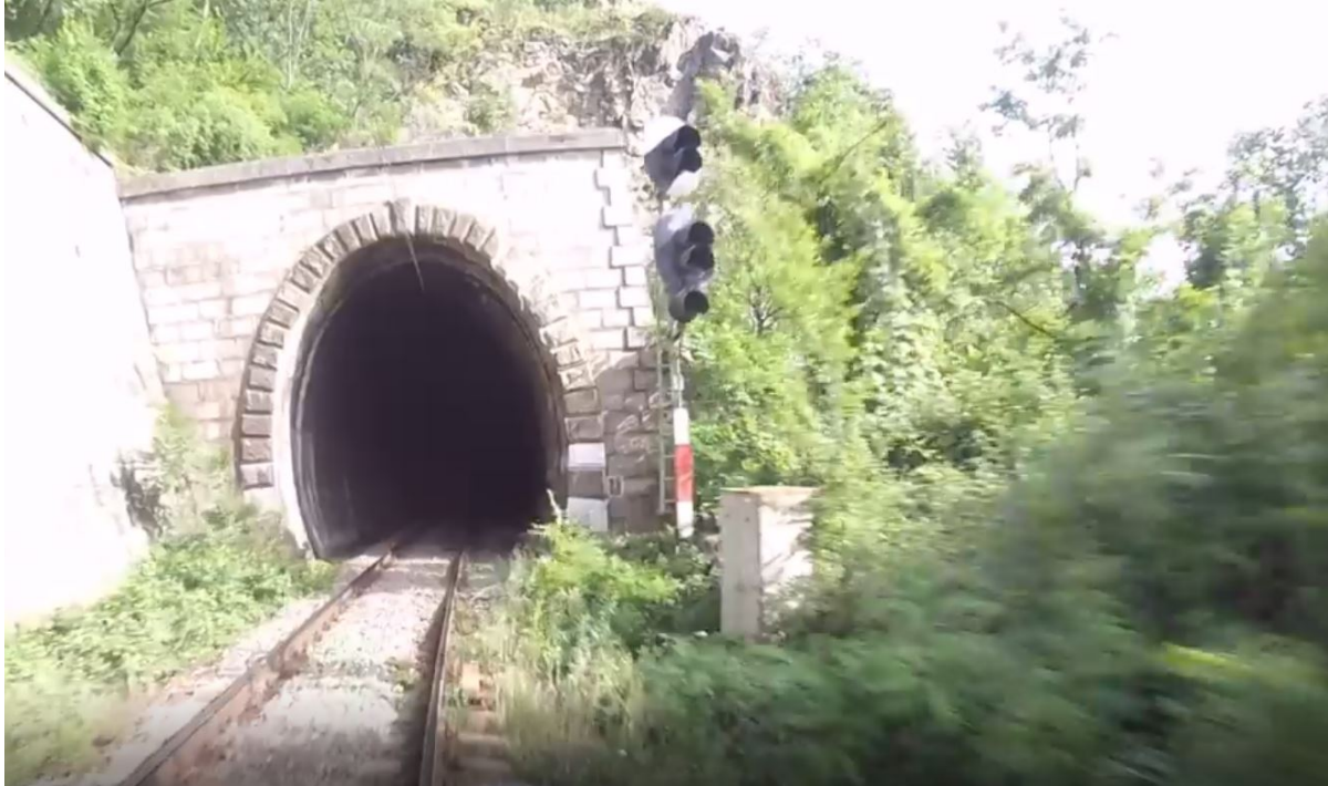
Figura 12: Tunel Tufari existent
