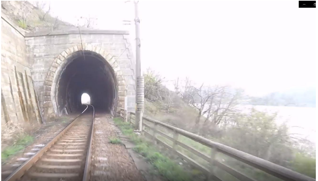
Figura 31: Tunel Vircirova existent
