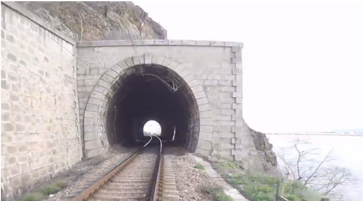
Figura 27: Tunel Baba existent
