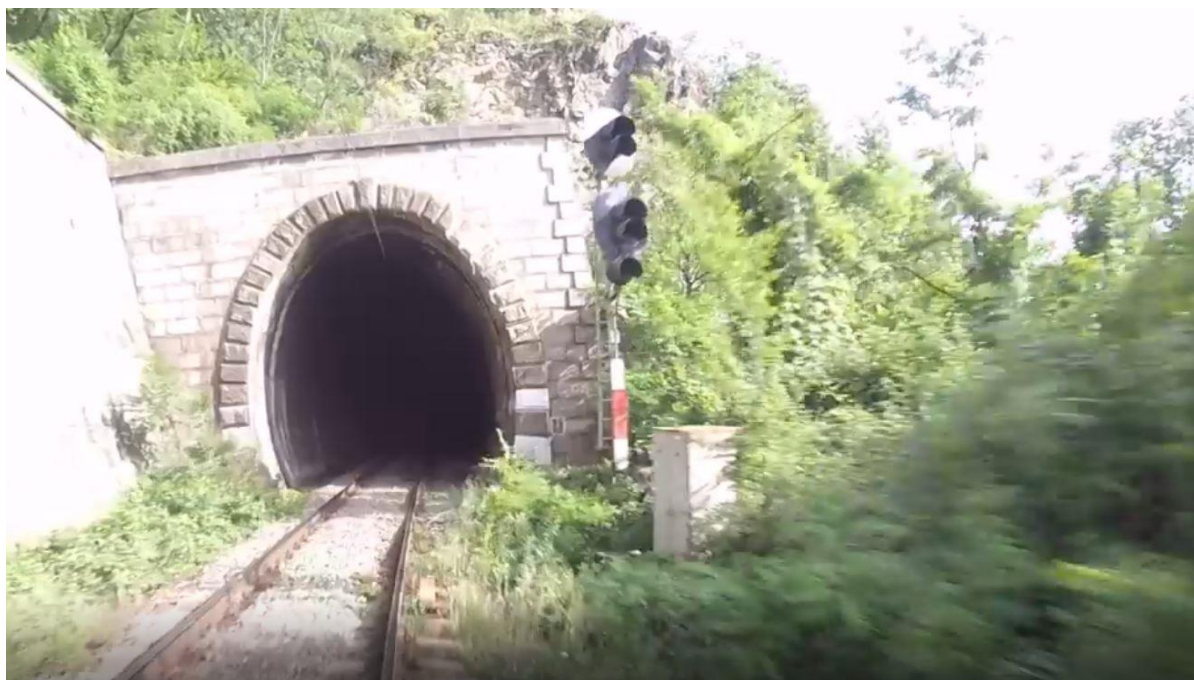
Figura 36: Tunel Tufari existent
