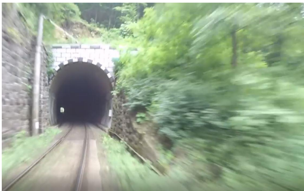
Figura 37: Tunel Rachitoberg existent
