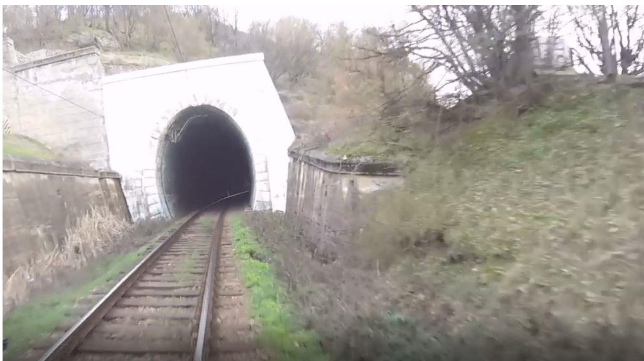
Figura 33: Tunel Bahna existent
